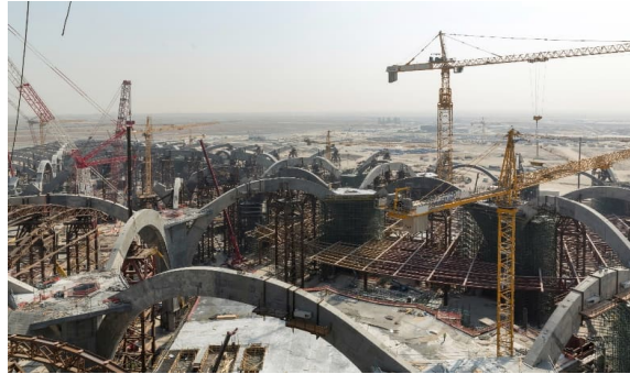
Roof Temporary Works 100.000tons
