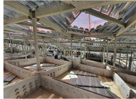
Roof Secondary Steelworks 18.000tons
